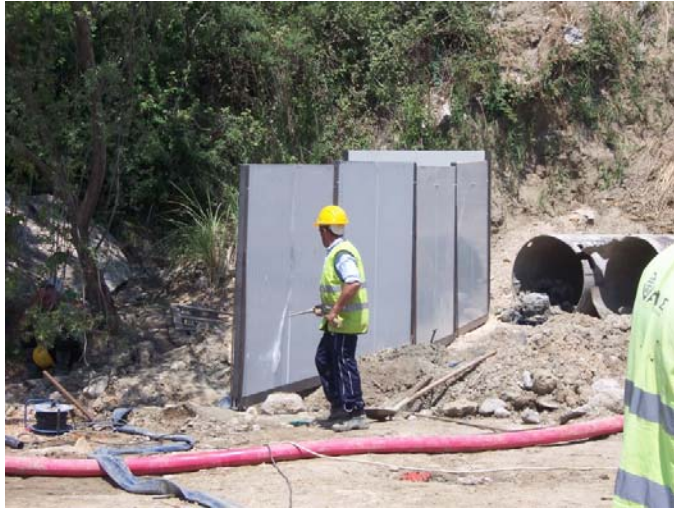
Superposition of movable noise barriers at the worksite of Sperhios river bridge (nea kiti - CH. 4+560 approximately)
