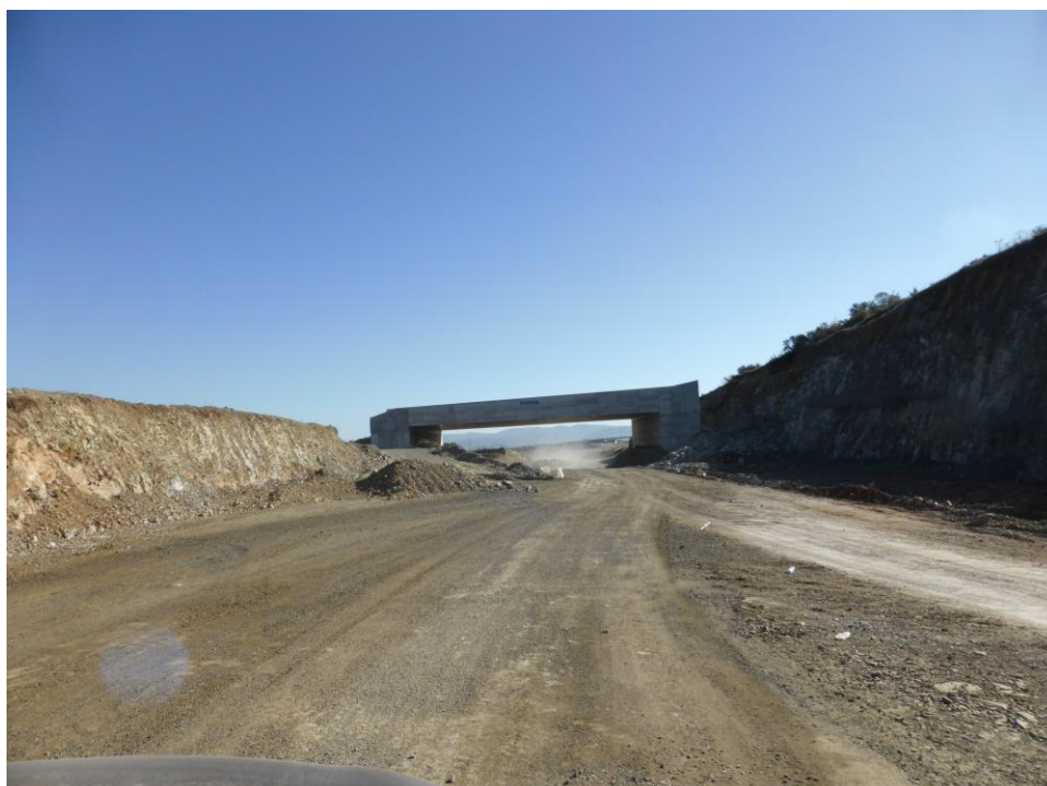
Under-construction of Fauna Upper-Pass (Green Bridge), of a width of 30m, at CH. 43+856,
