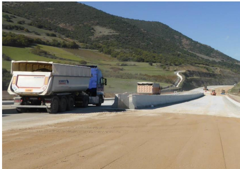
Transportation of loose earth materials with trucks equipped with the necessary equipment to reduce dust ("curtains", mudguards, blast pipes facing away from the ground).
