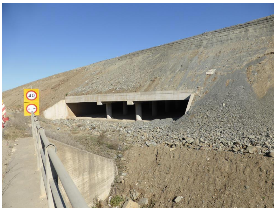
Construction of Fauna Under-Pass, of dimensions of 25,5X4,5m., at CH. 46+937, by order of the fauna monitoring program. The works of the openings final configuration still remain.
