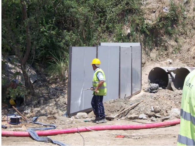
Photo 1. Superposition of movable noise barriers at the worksite of Sperhios river bridge (nea kiti - CH. 4+560 approximately)
