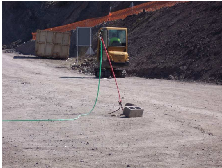
Photo 1. Installed semi-permanent sprinkler for the worksite at T2 in order to reduce dust emission
