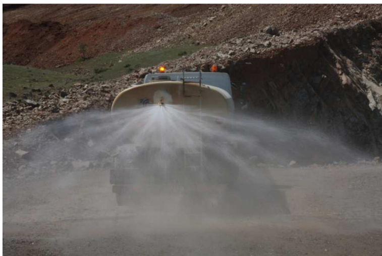
Photo 2. Systematic springing of the worksites in order to reduce dust
